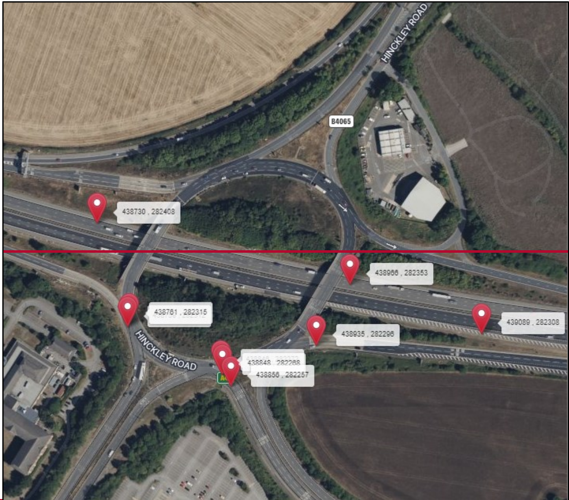
Figure 3.6: M6 Junction 2 Roundabout
