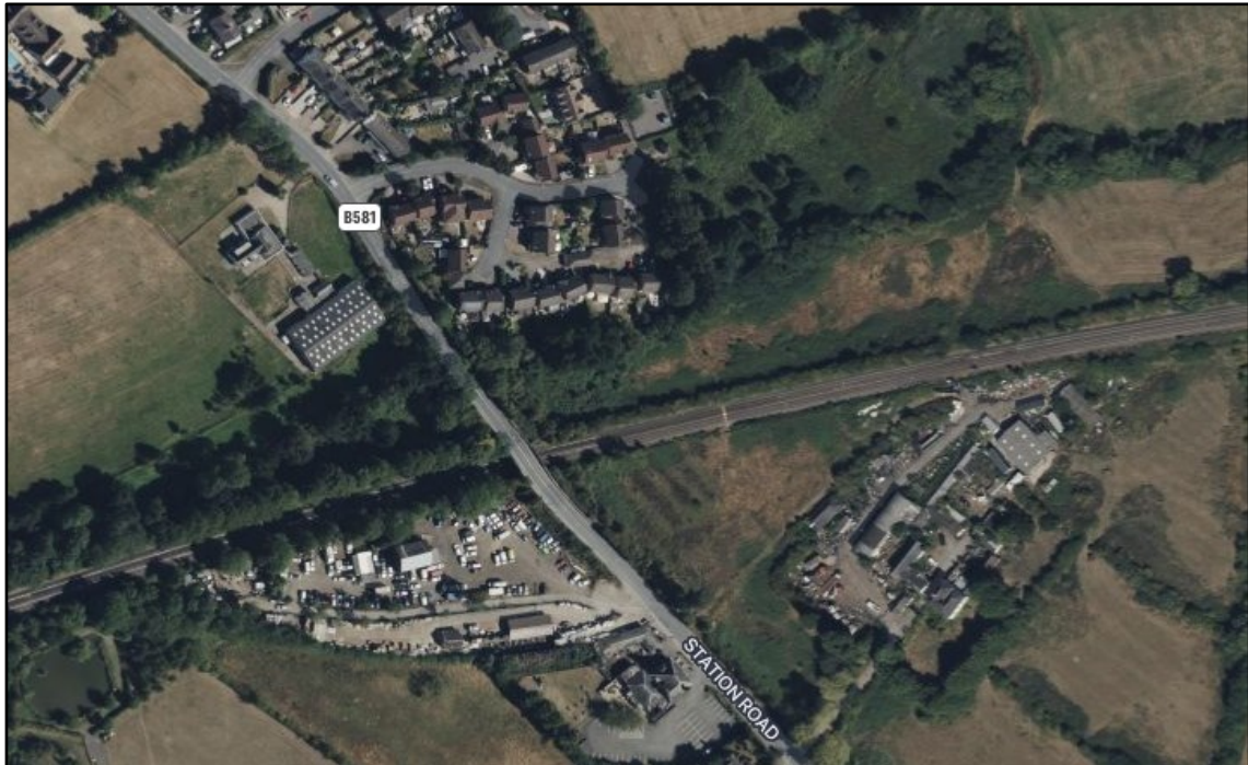
Figure 2.12. Station Road Railway Overbridge Elmesthorpe
