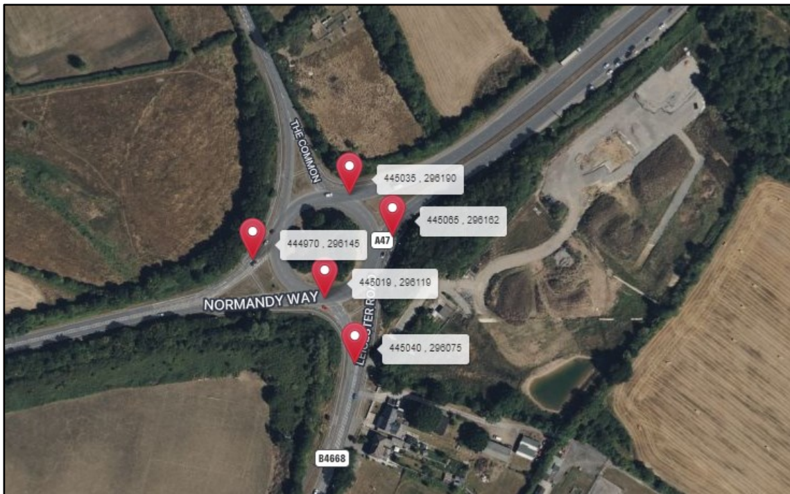
Figure 2.6: A47 Normandy Way/A47 Leicester Road/Road junction
